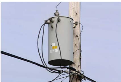
Pole Mount Transformer
